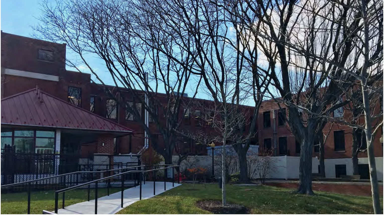
25,000 sq.ft. Office Building
