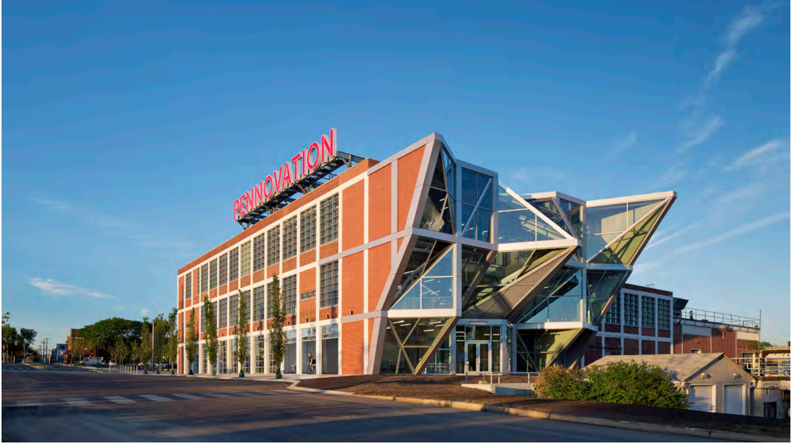
East and north facades
