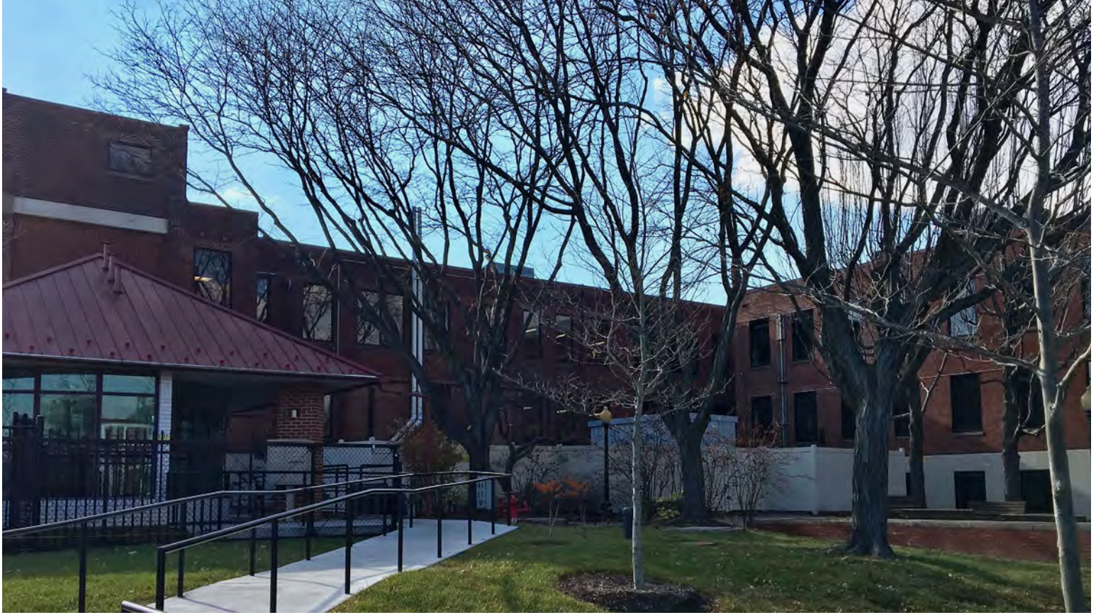
25,000 sq.ft. Office Building
